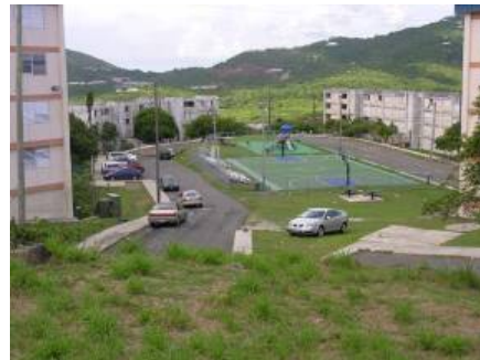
Looking toward Buildings 1 and 9
